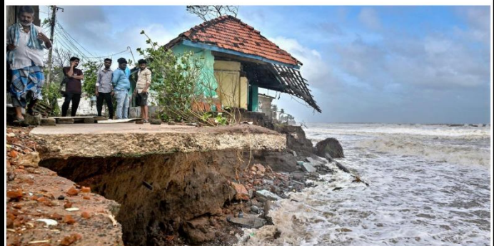
Swept away: A home destroyed by the cyclonic swell in Kakinada district of Andhra Pradesh on Tuesday. K.R. DEEPAK
