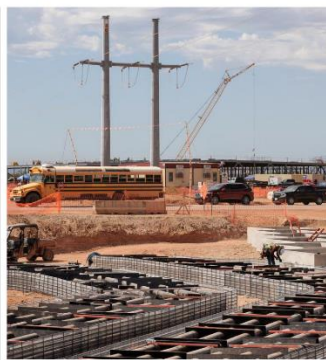
The future: Superclusters of data centres under construction in Texas, U.S., on September 23, 2023.
