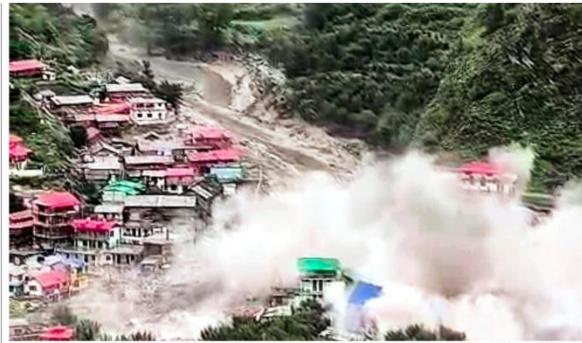
A screenshot shows houses being swept away after heavy rains triggered by a cloudburst at Dharali, Uttarakhand district, Uttarakhand in August 2025. PTI
