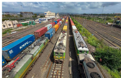
Infra boost: The Western Dedicated Freight Corridor (WDFC), virtually inaugurated by PM Narendra Modi. PTI
